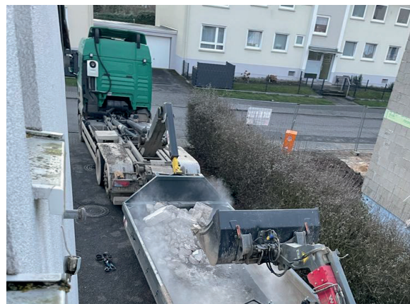
Disposal of construction debris using telescopic loaders
