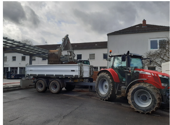
Transport of construction debris, mud, and other debris using earthmoving buckets
