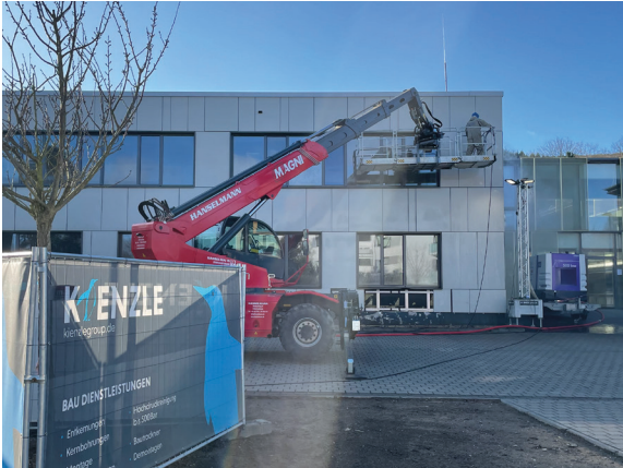
With the telescopic loader, work at heights of up to 21 meters is possible
